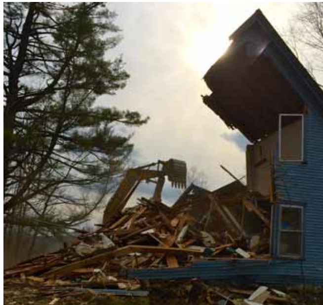
Demolition Day, November 5, 2014
